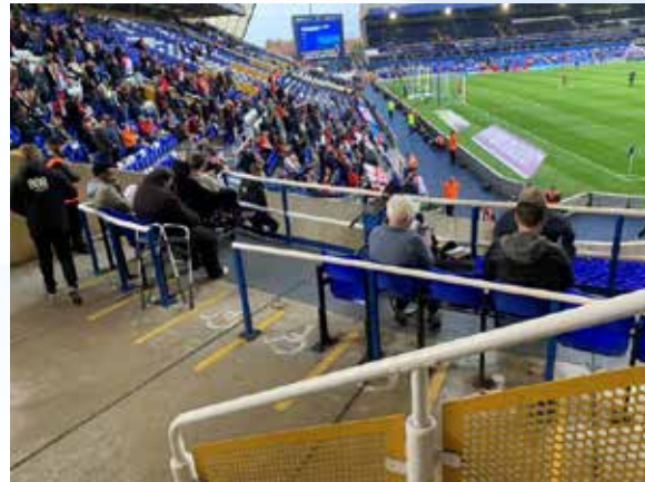
Wheelchair bay located in the KOP Stand
