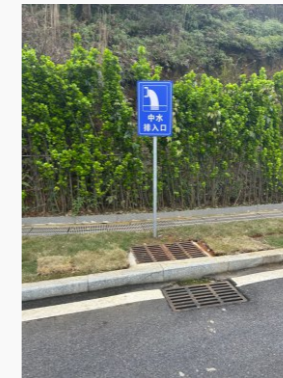
Winery Phase I Wastewater Station Reclaimed Water Reuse Project
