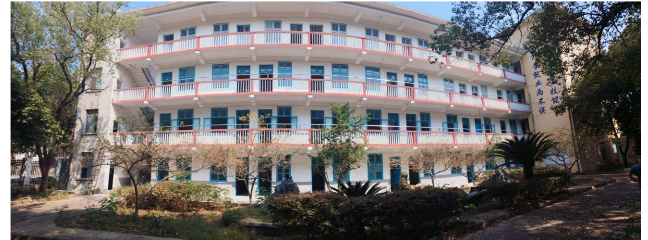
Employee Dormitory Upgrades
