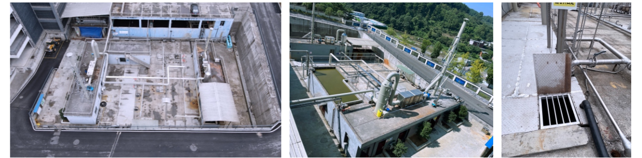
Closed renovation of sewage treatment station
