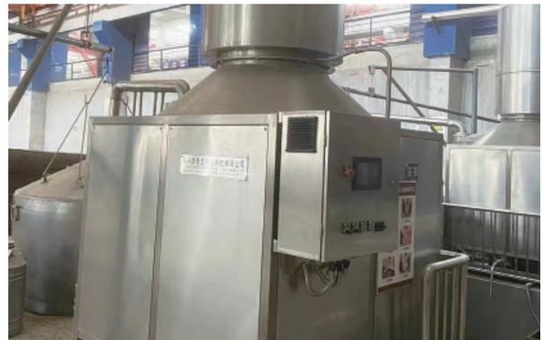
*Replaced the water-cooling system by air-cooling*
