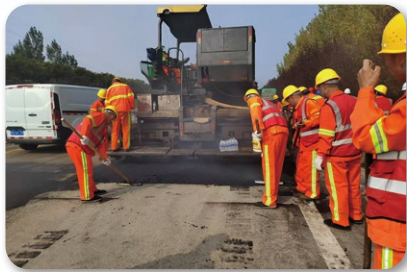
The new technology of low-carbon ultra-tough thin layer with a thickness of 1.5 cm is being used for construction
