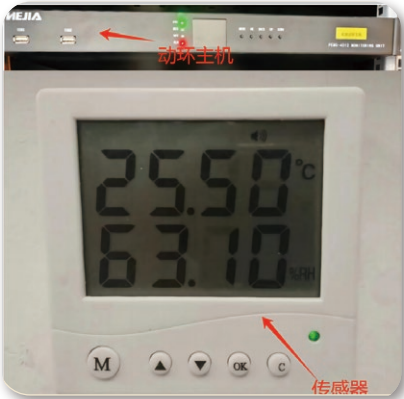
Temperature and Humidity Sensors Installation
