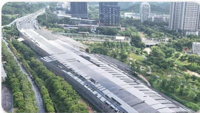
Aerial photo of the steel structure construction site of China's first fully enclosed sound barrier built on an existing ten-lane highway: The fully enclosed sound barrier construction project at the Baoli-Luolan Community section of the GNSR Expressway
