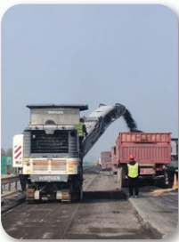
Deck milling of Shahe Bridge
