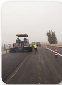
The top paving site of Shahe Bridge
