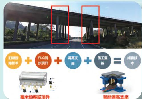
The inverted L pier replacement scheme of overall widening is adopted for the main line bridge of GNSR Expressway undercrossing China South Expressway
