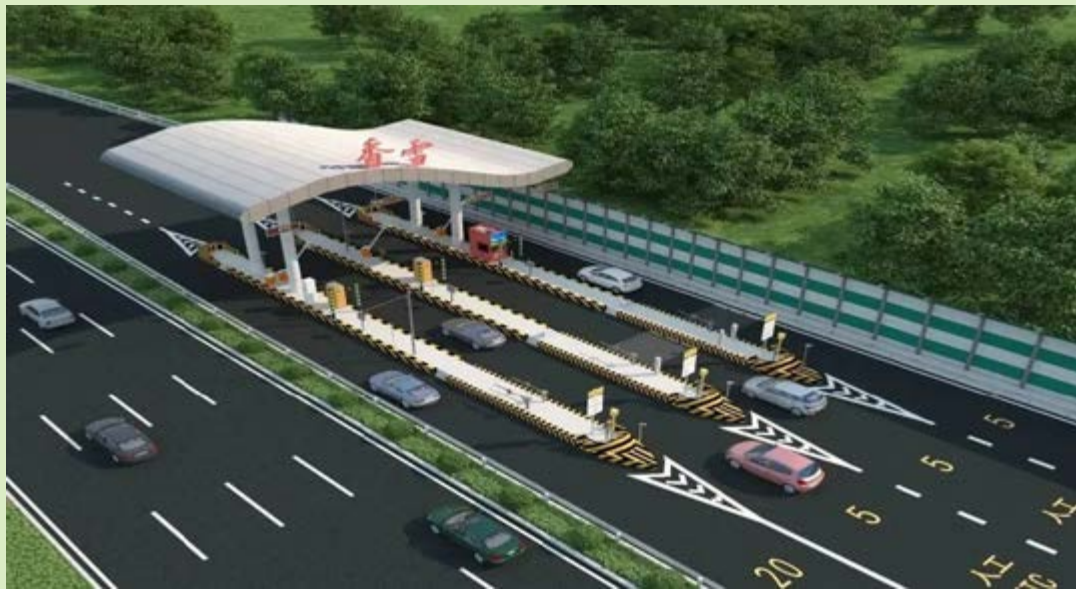
Guangzhou Xiangxue Unmanned Toll Station
