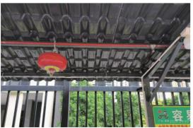
Equipped with water-based fire extinguisher
