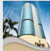
City Development Plaza (城建大廈)
