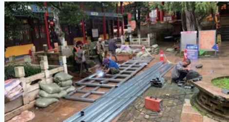
Framework Platform Welding
