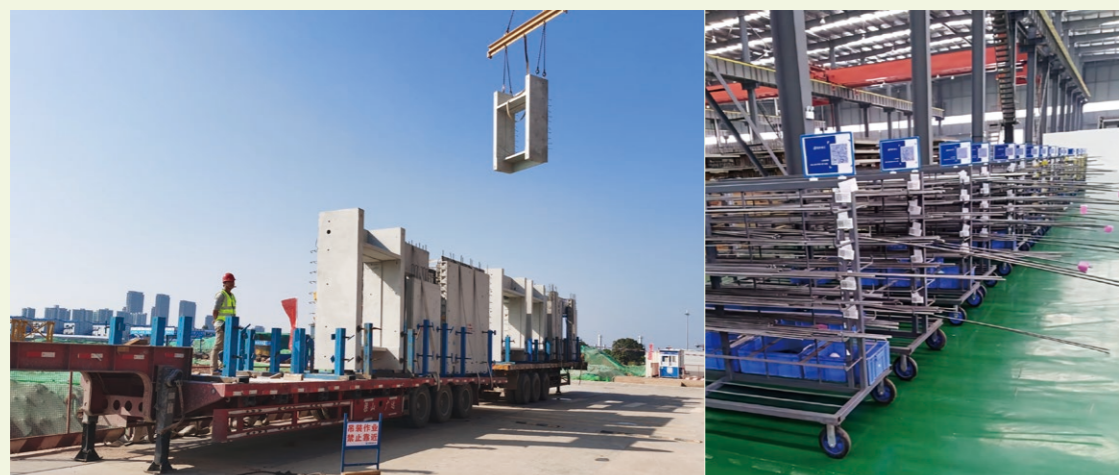
Processing Factory of Prefabricated Construction
