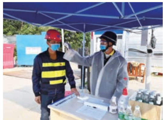
Temperature check conducted on the staff before access to the construction site
