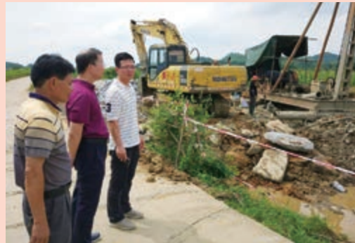
Checking the Construction Progress of Chimi Bridge
