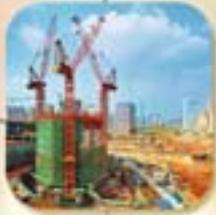
First lifting of the climbing formwork system of the main tower
