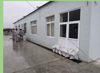
Reinforcing the camp
