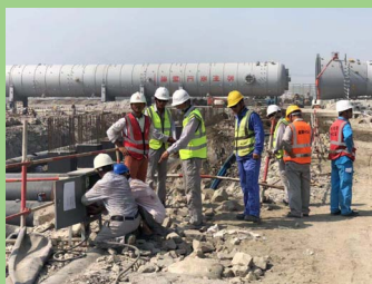
Camp inspection by the construction company (1)
