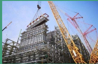
Modular installation of cracking furnace
