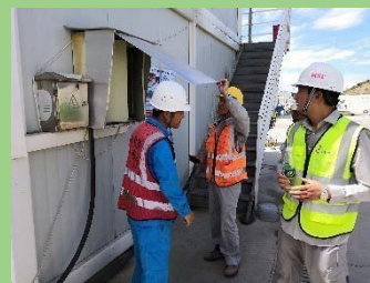
Camp inspection by the construction company (2)
