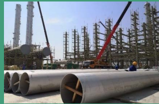
Soilless construction of pipeline
