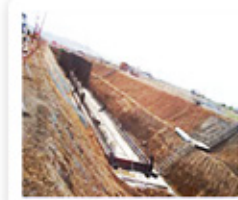
Operation under ground
