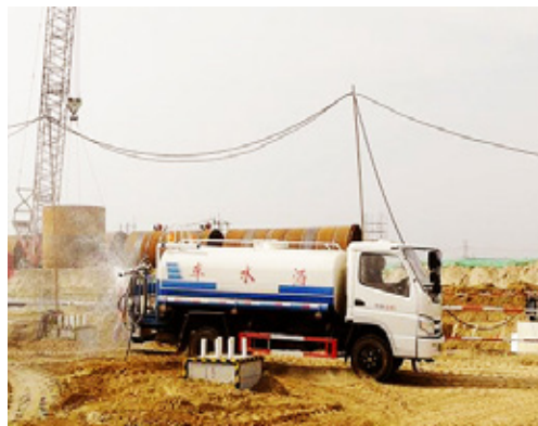
Spraying water for dust control
