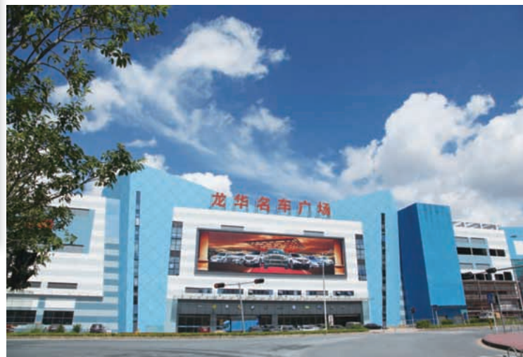
▼ New Logistic Centre at South China Logistic Park
