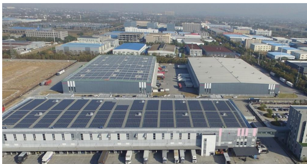
To support the use of renewable energy, SF REIT has installed solar panels at the rooftop of its properties.
