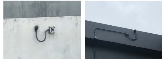
Light sensors at the rooftop and 9/F of the Tsing Yi Property
