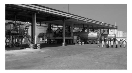
This picture shows trucks loading products at station via pipes connected to storage tanks.
