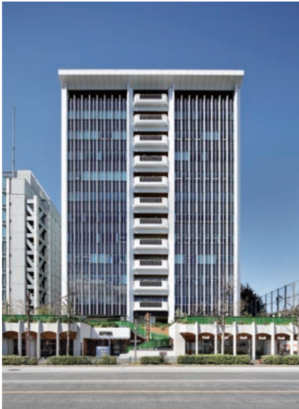
Aoyama Building, Japan
