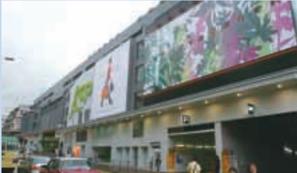
New Facade, KCP, Kowloon City
