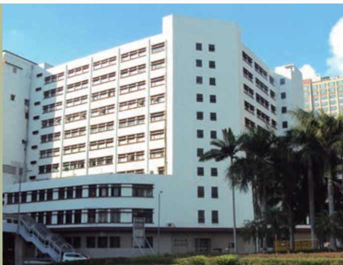
Pioneer Building Elevation – before conversion
