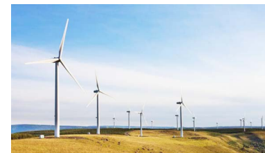
Onshore wind power in Xiqing District, Tianjin
