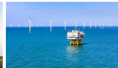
Rudong Lugu offshore wind power in Jiangsu
