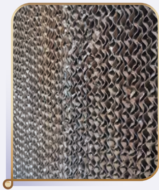
Warm air is pulled through the water-saturated pads, causing the water to evaporate and cool the air inside Central Laundry.
