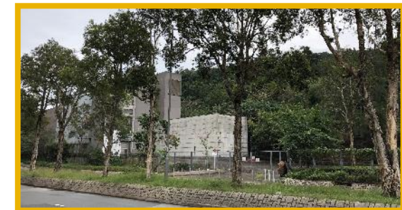
Pak Shing Kok Ventilation Building
