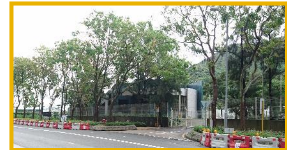
Tung Chung Traction Substation
