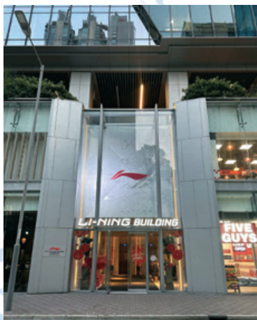
Hong Kong Li-Ning Building
