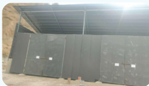
Photo: Garbage sorting warehouse of Full Gold
