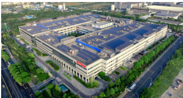
The image is of the solar panel installations at Lenovo's Wuhan, China location.
