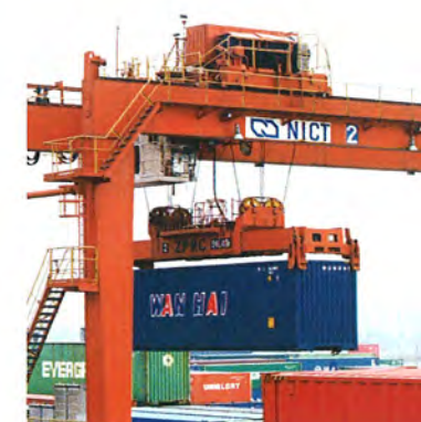
Nanhai International Container Terminals is one of the river ports of Hutchison Delta Ports.
