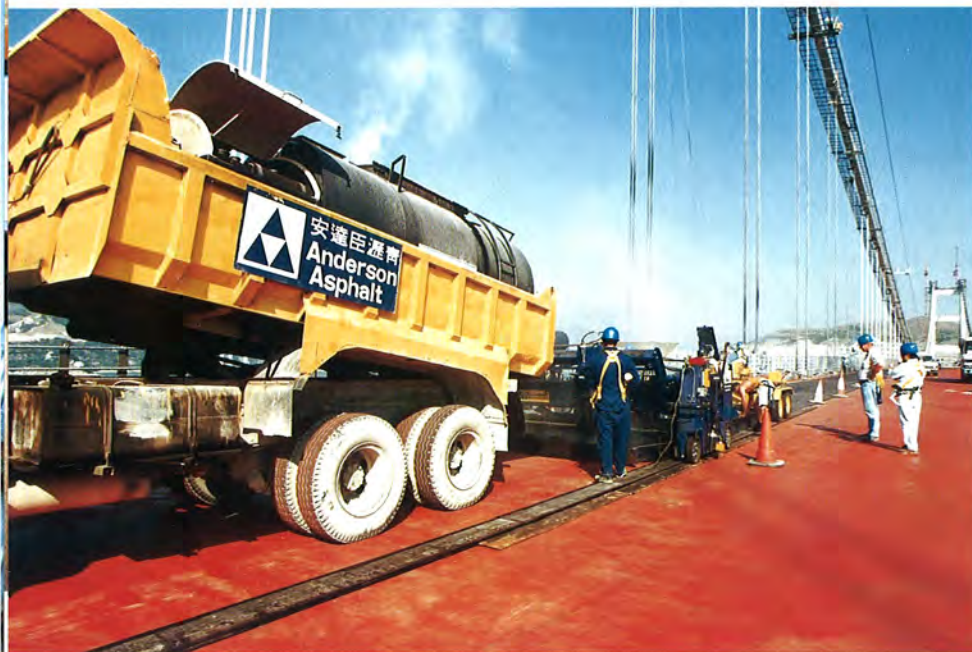
Mastic asphalt was laid on the deck of the Tsing Ma Bridge in Hong Kong.
