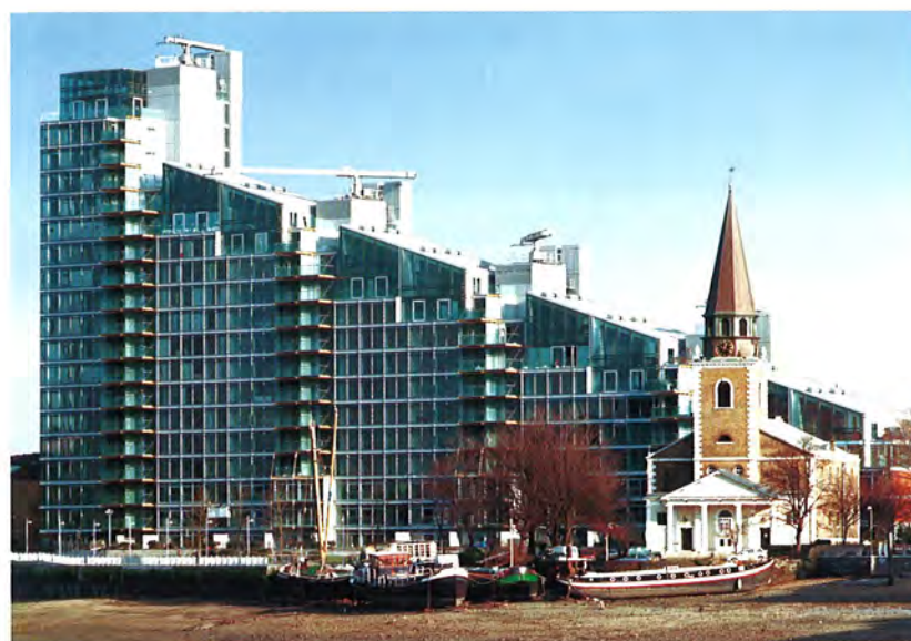
Situated at Battersea, London, Montevetro is an upscale residential complex commanding a spectacular view of River Thames.
