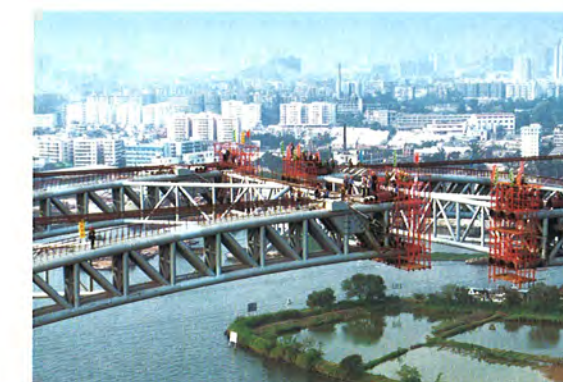
Advanced engineering and construction technologies were applied in the construction of the Ya Ji Sha Bridge.
