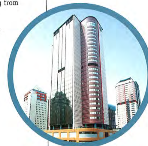
Harbour Plaza Chongqing has the advantage of its proximity to the airport and railway station.
