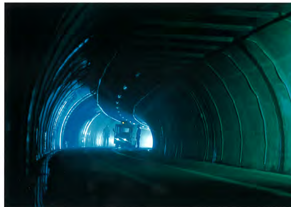
The Nam Fung-Parker Cable Tunnel, the second cable tunnel in Hongkong Electric's transmission system, is 5.7 km long.
