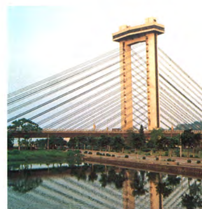
Comprising 11 roads and bridges, the Nanhai Road Network forms an integral part of the city's transportation system. This is the Nanhai Xiqiao Bridge.
