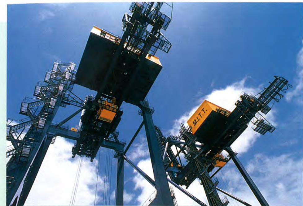
Myanmar International Terminals Thilawa has berthing capacity for four ocean going size vessels and a current capacity of 100,000 TEUs per year.
