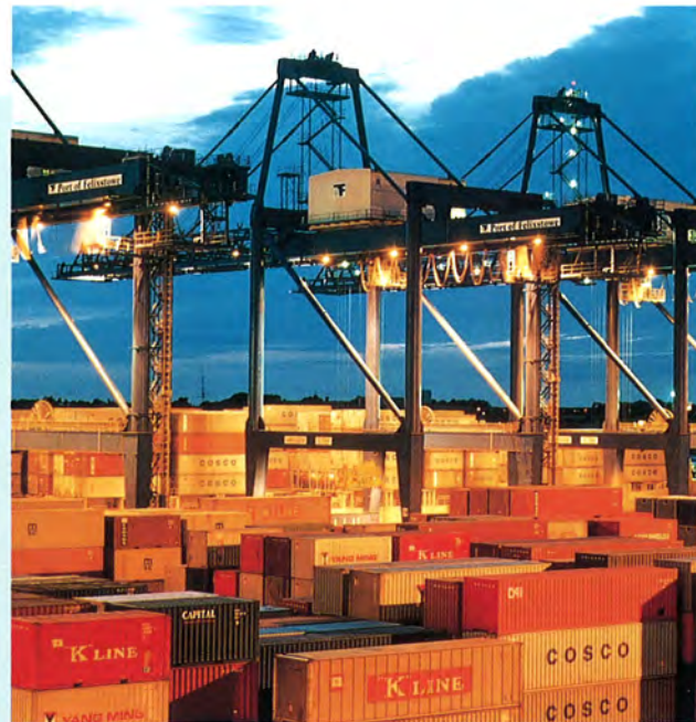
The £45 million investment in Trinity III will further enhance port efficiency and secure the Port of Felixstowe's position well into the millennium as the UK's largest container port.
