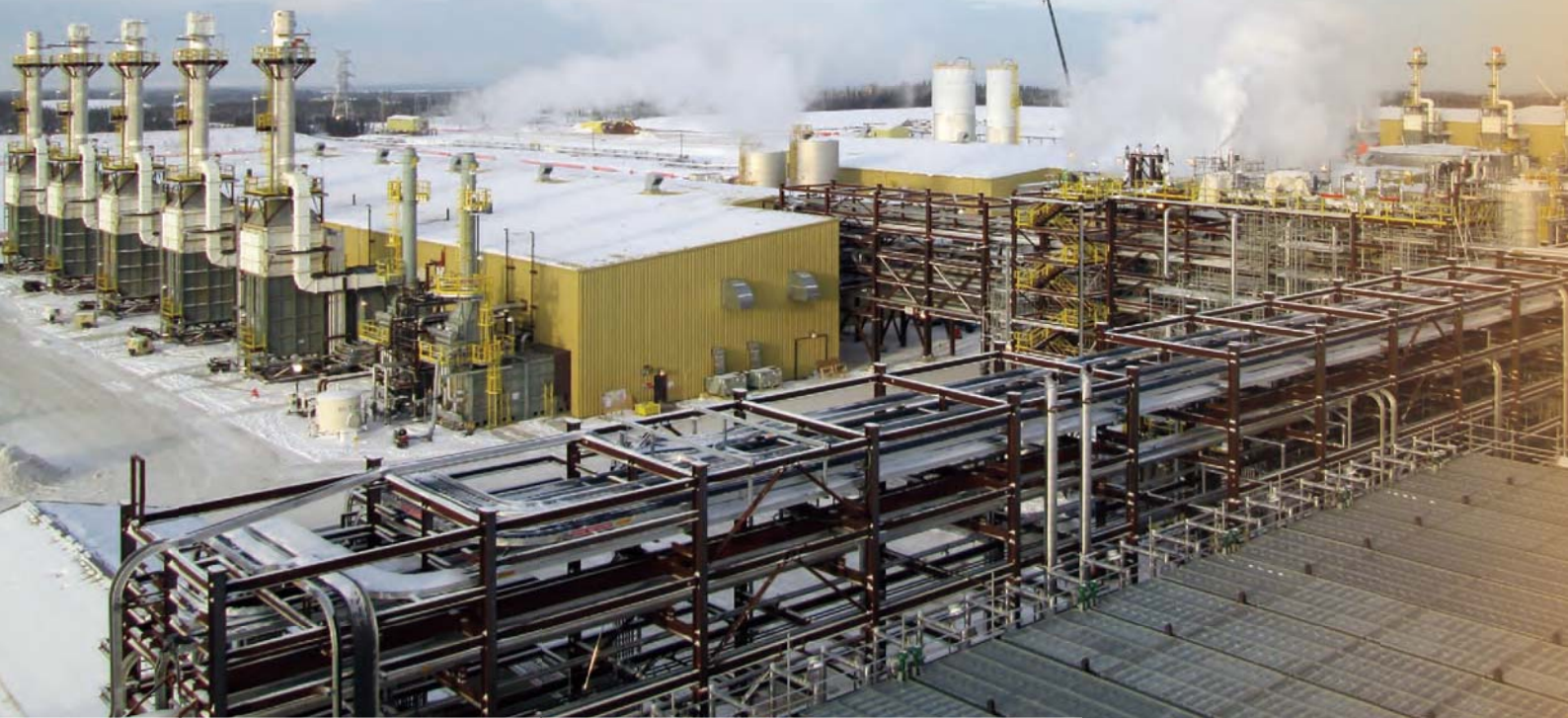
The Sunrise Energy Project commences steam operations.
