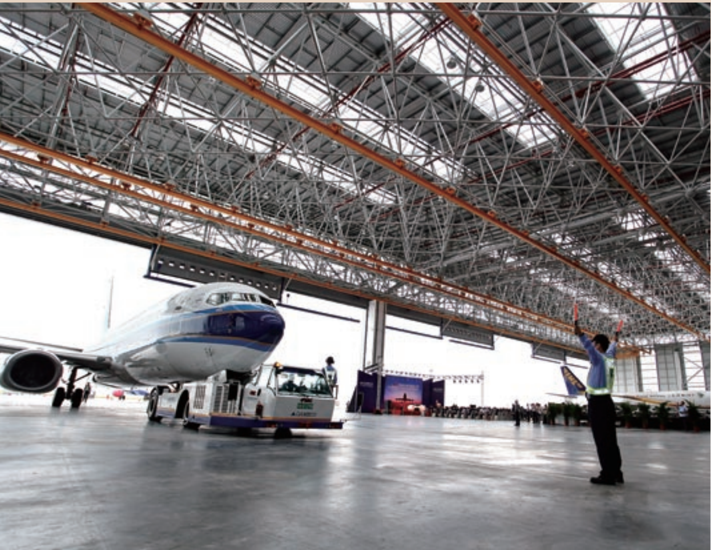
GAMECO announces the inauguration of the new Phase II Hangar.
