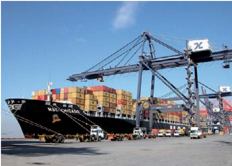
Xiamen International Container Terminals in Mainland China.
