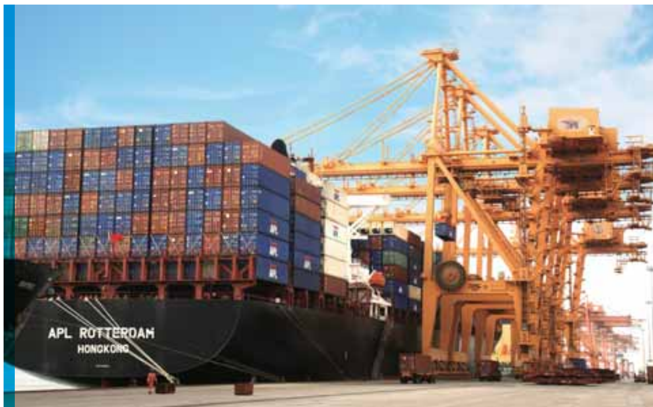
Quay cranes at International Ports Services, Dammam, Saudi Arabia, are servicing a container vessel.
