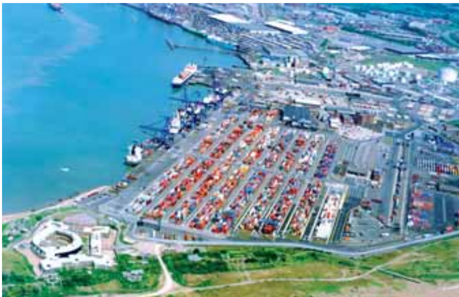
The Port of Felixstowe's South Reconfiguration will provide the United Kingdom with additional port capacity.
