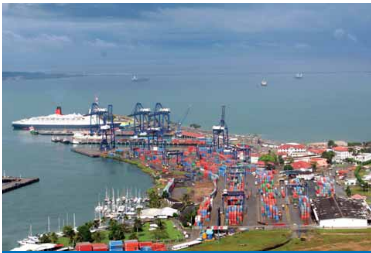
● Panama Ports Company – Port of Cristobal.
