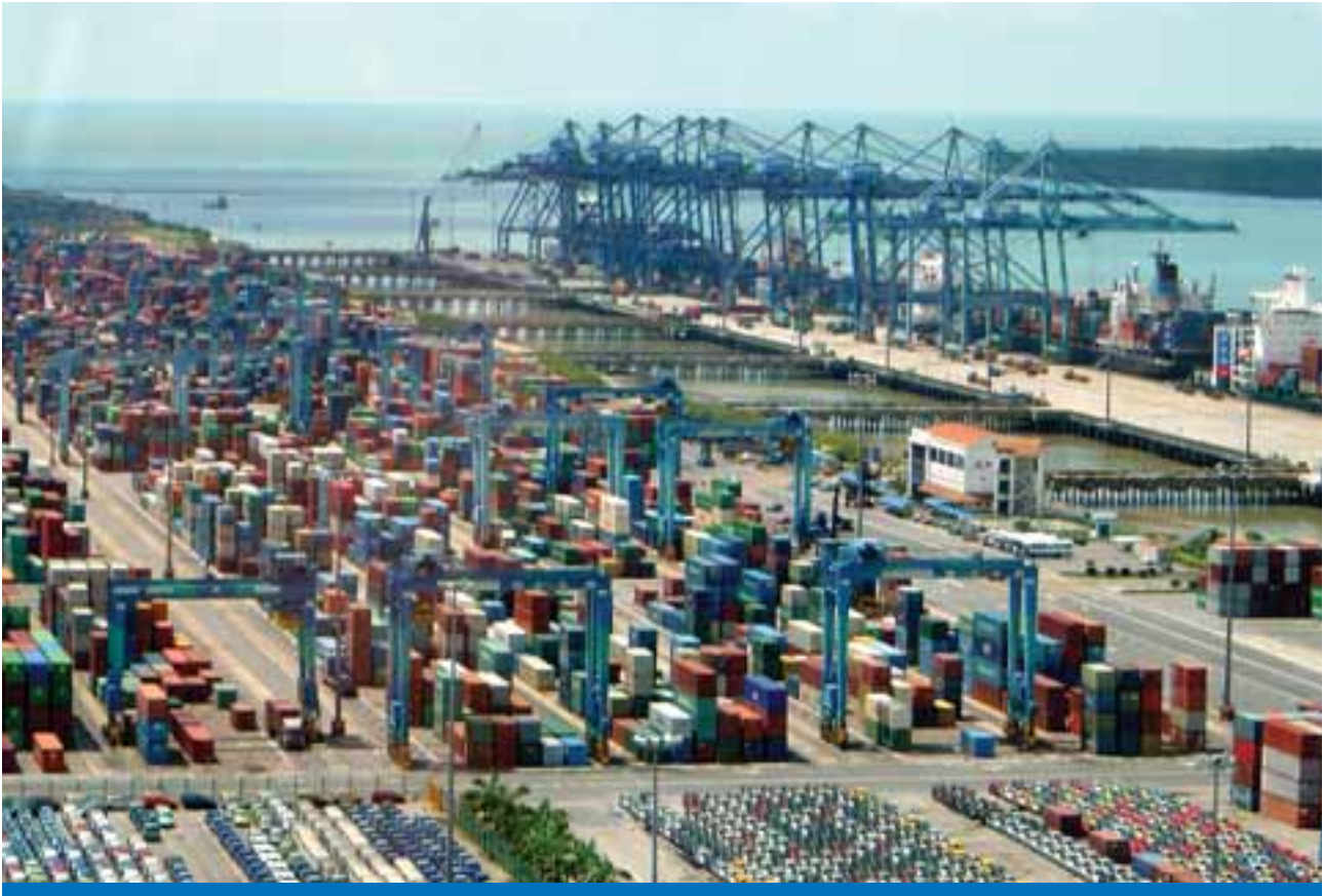
● The quayside and yard operations at Westports Malaysia.
