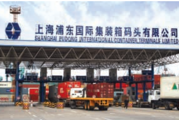
■ Shanghai Pudong International Container Terminals operates three berths at Phase I of the Waigaoqiao Terminal.
