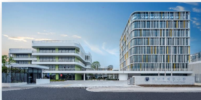
Diversified urban services Hangzhou Silicon Valley Primary School
