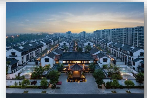
Capital owner projects Changzhou Jiangnan Lane
