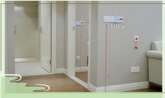
Setting the switch height to 110cm
