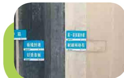
Construction method for interior wall: hollowing and cracks are effectively controlled by using lightweight panels of autoclaved ceramsite concrete for partition wall.
