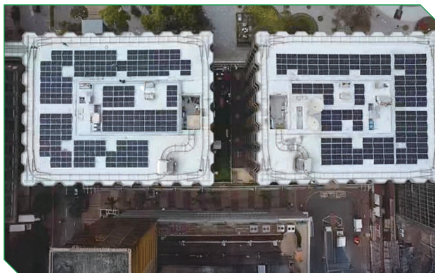
■ The rooftop solar energy facilities at the South Seas Centre in Tsim Sha Tsui, Kowloon, commenced grid-connected power generation in February 2024. It has a designed installed capacity of 194 kW and is the Group's 13th solar energy project in Hong Kong.
