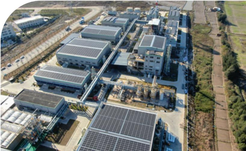
Wenling Solid Waste Treatment Project has constructed solar energy facilities at locations such as rooftops of the plant buildings, accident pools, preliminary rainwater captures with an installed area of approximately 12,000 m<sup>2</sup>, and an aggregate installed capacity of approximately 1.6MW.
