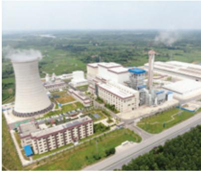
Built on a site area of 215 mu. Phase I of the household waste-to-energy project equipped with a mechanical grate furnace and a condensing turbine generator unit with a designed daily waste processing capacity of 400 MT and annual designed on-grid power generation volume of 47 million KWh to realise the reduction, recycling and detoxification of household waste and convert waste into value.
