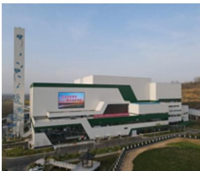
Located at the west side of Xiaomopan Hill in Liuhe District, Nanjing, the project offers a daily household waste processing capacity of 1,000 MT and an ash landfill with a capacity of approximately 350,000 cubic metres. Fume purification process technologies adopted include in-boiler deNO<sub>x</sub>, ex-boiler catalytic reduction deNO<sub>x</sub>, semi-dry deacidification, active carbon spray, dry-spray deacidification and dust removal bag.
