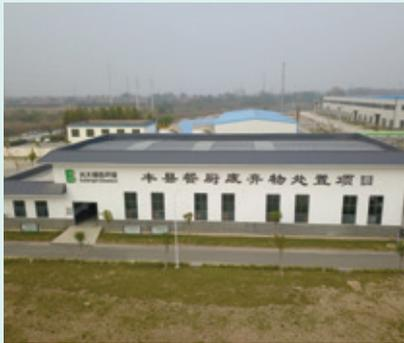
Built on a total site area of 98.25 mu, the project collects materials and puts them through processes such as macro-substance sorting, high-temperature steam cooking, solid-liquid separation, pyrolytic oil extraction and residue incineration. The integrated kitchen waste treatment workshop is a concealed operation where odour is incinerated once and for all in the inhouse waste incinerator after collection. The project has a daily kitchen waste processing capacity of 60 MT.
