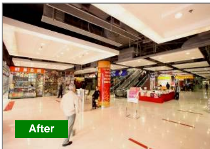
New ceiling, lighting and flooring
