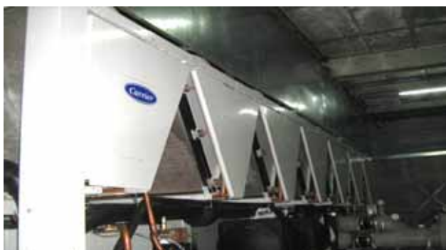
New replacement of Air-conditioning chiller
