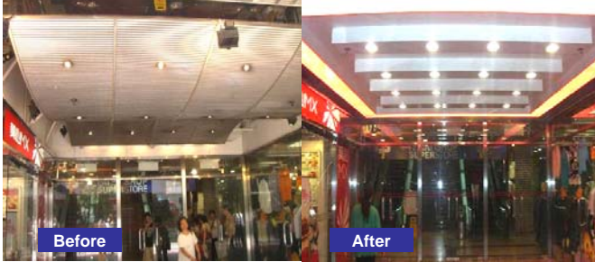
Smartland: Upgrading of ceiling and flooring
