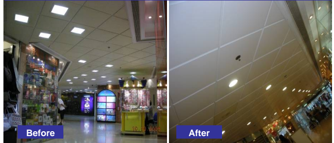
Ma On Shan Plaza: Energy saving bulbs and ceiling upgrade
