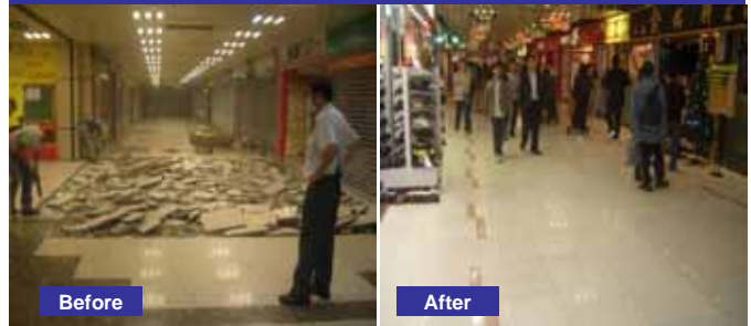
Waldorf: New floor tiles in main corridor
