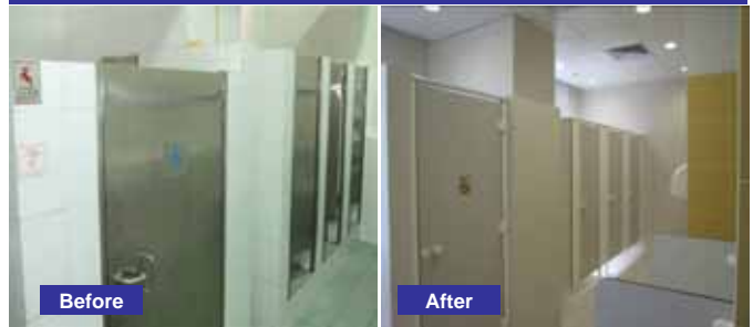
Waldorf: Upgrading of washroom
