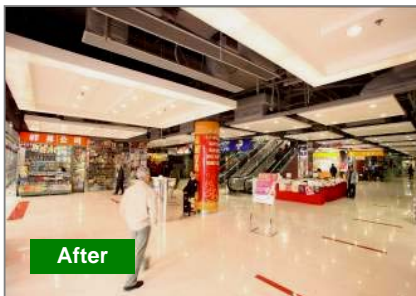
New ceiling, lighting and flooring
