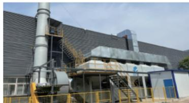
The Company has adopted activated carbon adsorption and desorption with catalytic combustion, and zeolite wheels with RTO technologies to improve the treatment of waste gases from painting processes, thereby reducing the emission of waste gas pollutants. Anemometers have been purchased to measure wind speed and direction around production equipment, standardizing the monitoring of unorganized emissions from painting waste gases, and meeting government industrial pollution control requirements.
